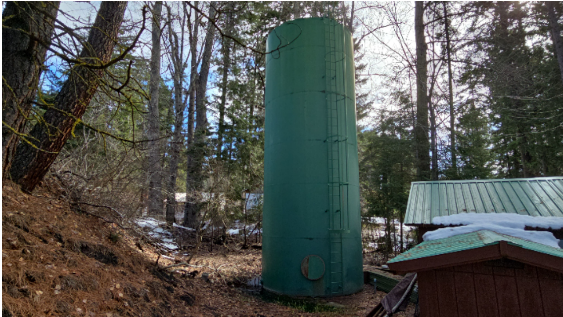
General Site - Station 2, Tank, 30,000 Gal.
